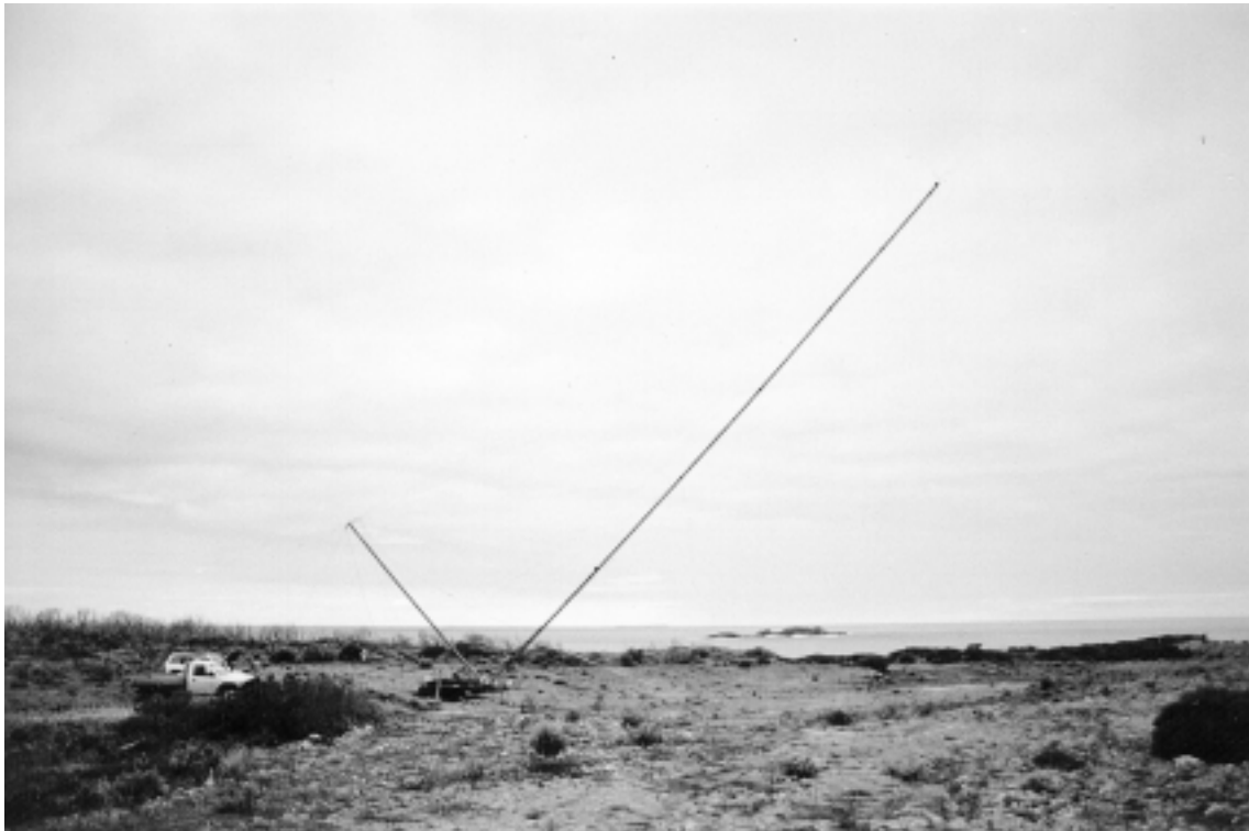
Figure 5 – Erecting 45m Pole Mast with Winch and Gin Pole (courtesy Enviromet Meteorological Consultants)
