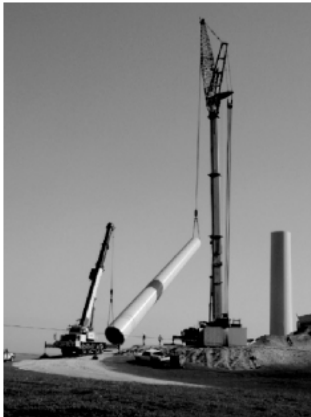
Figure 15 Codrington Lower Tower Section Lift (courtesy Pacific Hydro)
